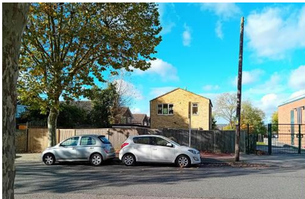
Figure 3 – Front elevation of School House
